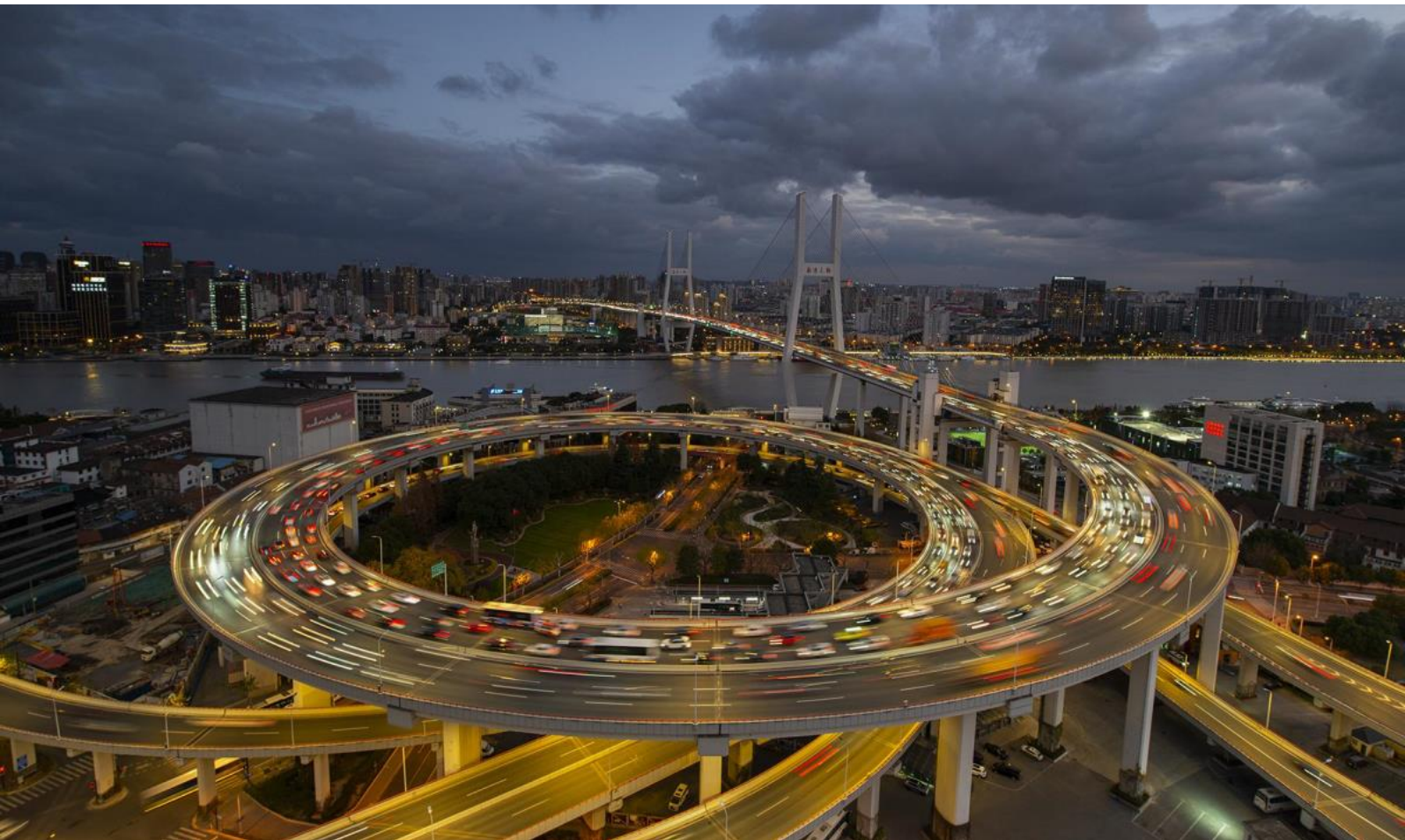
GPU HM - NANPU BRIDGE 13 by ZHICAI REN (CHINA)
